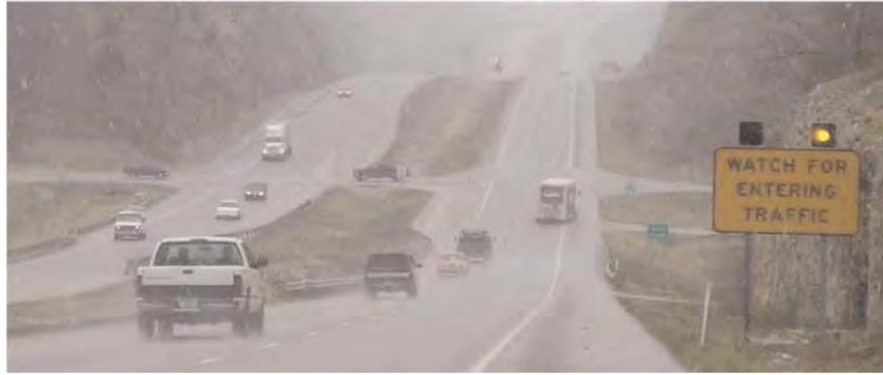
Figure 7.3.1: Example of a Dynamic Advance Intersection Warning System
