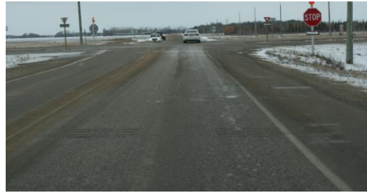
Rumble strips on the westbound approach
